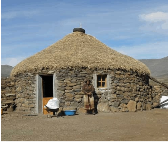
We visited this typical mountain home, her husband, built it from rocks and thatching grass. The roof is supported by tree poles brought from South Africa as no trees grow in the highlands.
