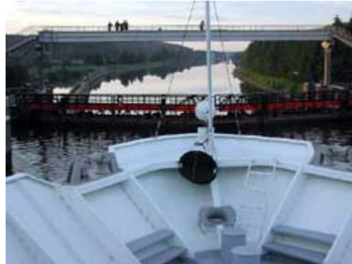
We pull into the first gate. After the water drains out, the boat is 8 meters lower and the gate opens. It is remarkable that the rear gate is brought up from the riverbed; the front gate swings open
