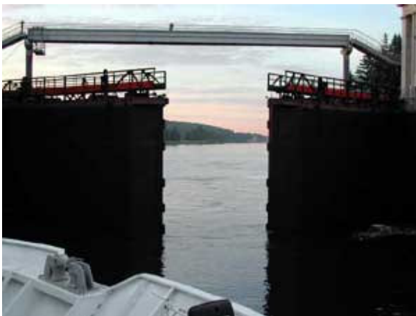
We pull into the first gate. After the water drains out, the boat is 8 meters lower and the gate opens. It is remarkable that the rear gate is brought up from the riverbed; the front gate swings open
